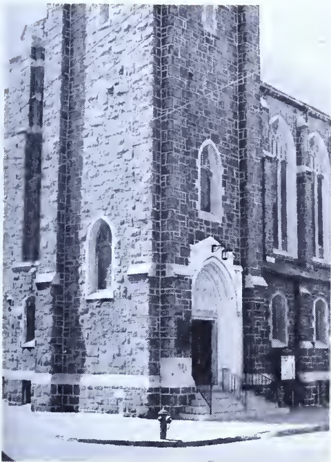
Christ Evangelical Lutheran Church, 124 South Thirteenth Street; granite from Seisholtzville, Berks County.
